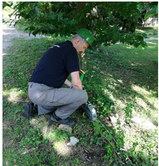
Figure 3.16. Feeding the cable into the winch
